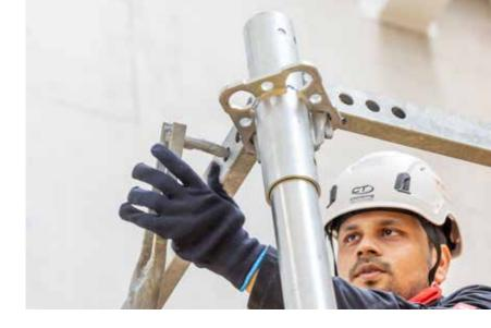
The PERI UP Shoring Tower MD is a versatile medium-duty shoring system designed specifically for infrastructure projects and building construction with thick slabs. The system's modular and flexible design, featuring Gravity Lock Technology, ensures simple and safe assembly.
