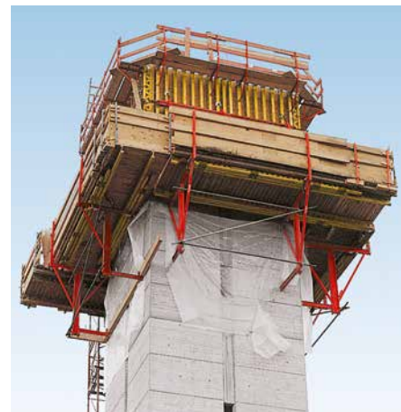
Church steeple in Feldmoching near Munich. VARIO GT 24 on KGF 240 climbing formwork.
