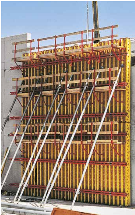
Extended VARIO GT 24 panels being used to shutter administration building.
