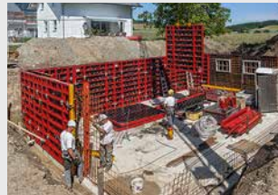
Wall Formwork
