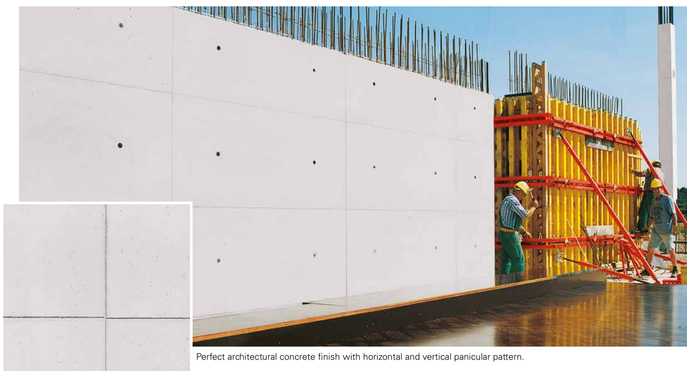
Consecration Hall, Neuburg, Germany. VARIO with an orderly tie pattern. Formlining screwed on from the rear.
