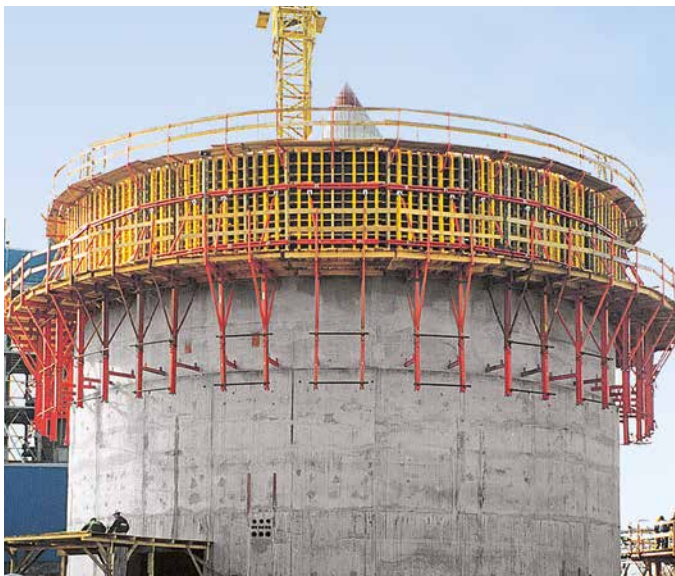
VARIO GT 24 being used to construct a circular tank. Timber wedges between girders and steel walers produce the circular shape.
