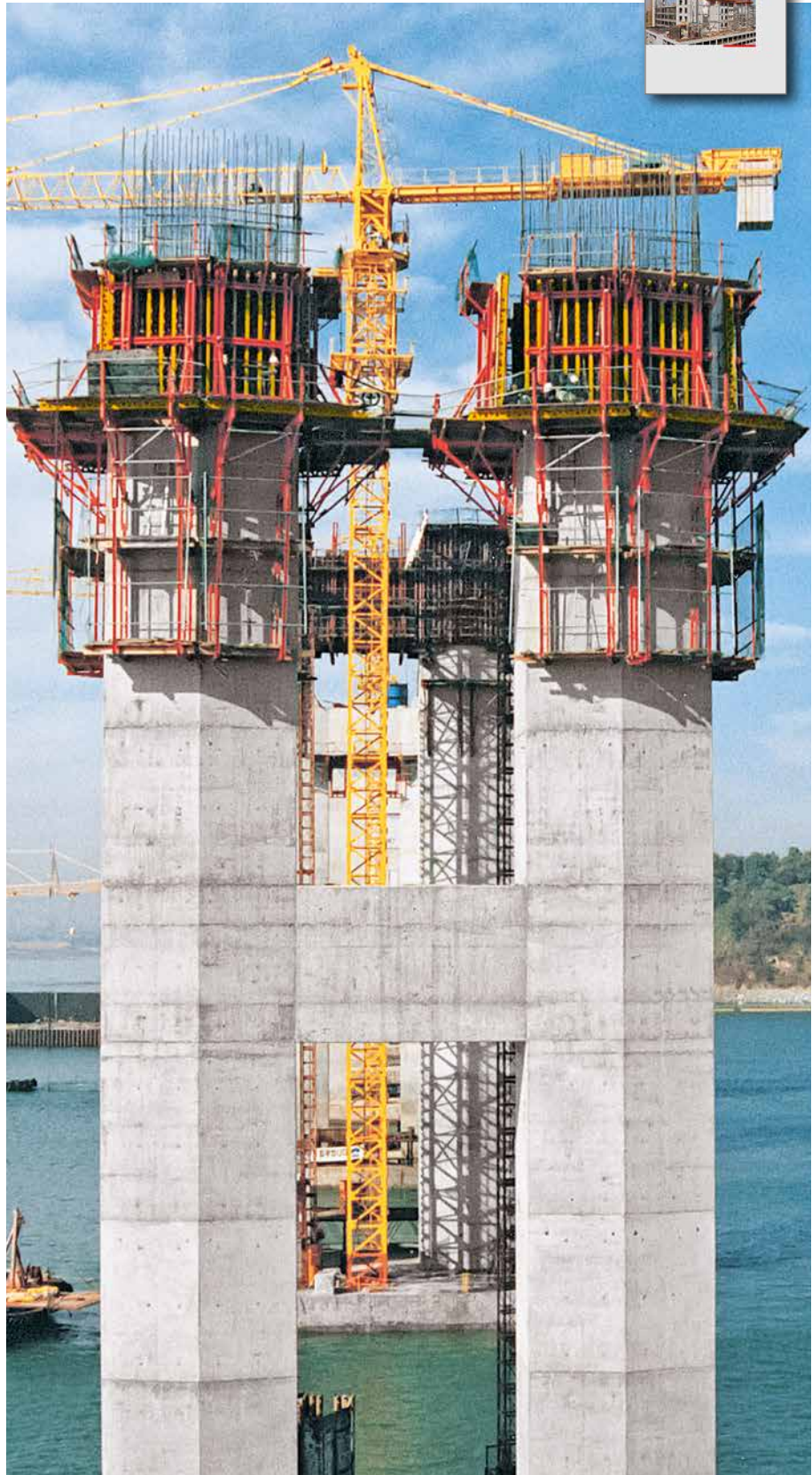
CB 240, the triangular bracket for problem-free working in front of and behind the formwork.
