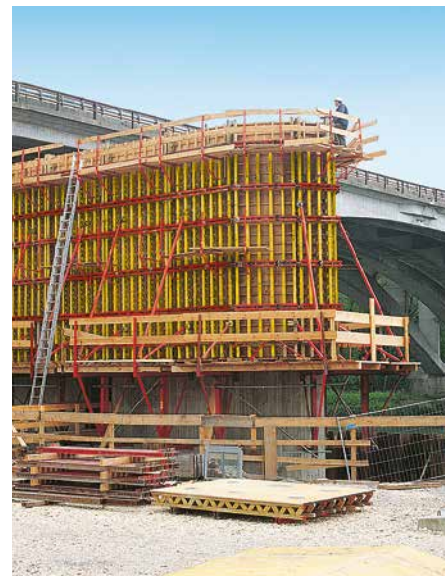
Sides of hollow piers on the banks of the river, climbed with VARIO GT 24 on PERI KG 240 climbing scaffold. Adapting to the arch-shaped ends was achieved with VARIO standard components and forming boards.
